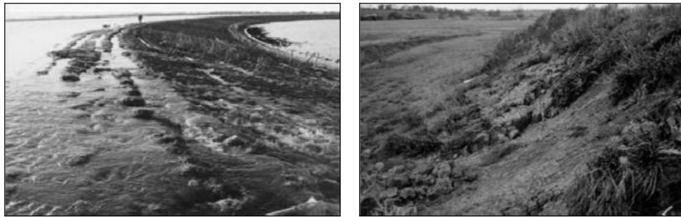
Figure 1. Embankment overflow protected by grass cover (Left); Wave overtopping erosion of a coastal embankment (Right) (Photos from the EU FLOODsite project)
